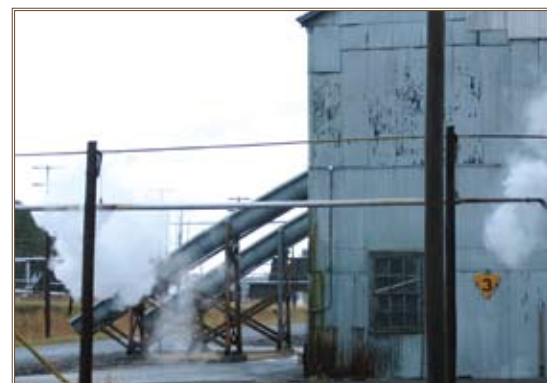
Leaking steam from distribution systems, like this one at Radford Army Ammunition Plant, Va., cause water use to rise. Photo courtesy of William Eng
