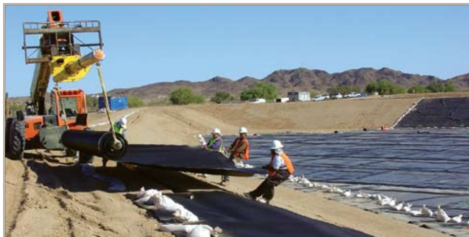
Construction crews roll out hundreds of feet of high-density polyethylene geomembrane lining at the sewage lagoons. Photos by Mary F. Flores
