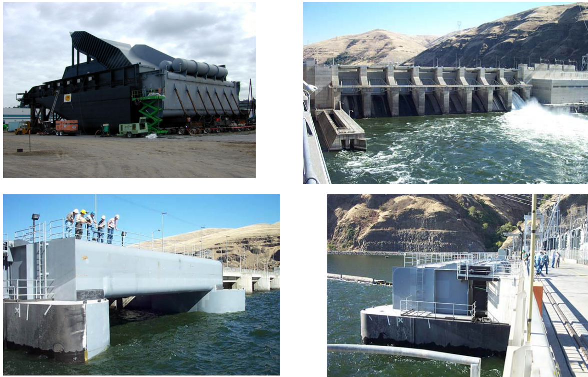
Figure 8. Photos of the Removable Spillway Weir at Lower Granite Dam. Counter clockwise, from upper left: RSW on land; forebay view of RSW in place; RSW in place, view from the dam; RSW spilling water at the right-hand spill bay. (Photos courtesy of U.S. Army Corps of Engineers)
