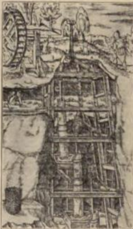
Fig. 15.—Early Application of Undershot Water Wheel to Mine Drainage. Date Unknown (from Cassiers Mag. March, 1899).
